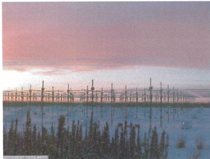
The HAARP-antenna array at Anchorage, Alaska 115
